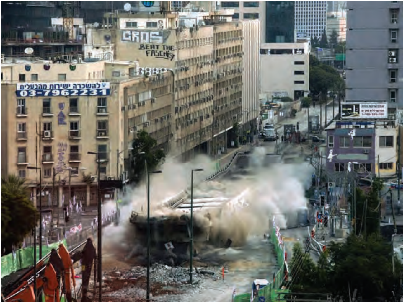
Demolition of the "Maariv" overpass to make way for the Tel-Aviv light railway station there and an underpass to replace it.
