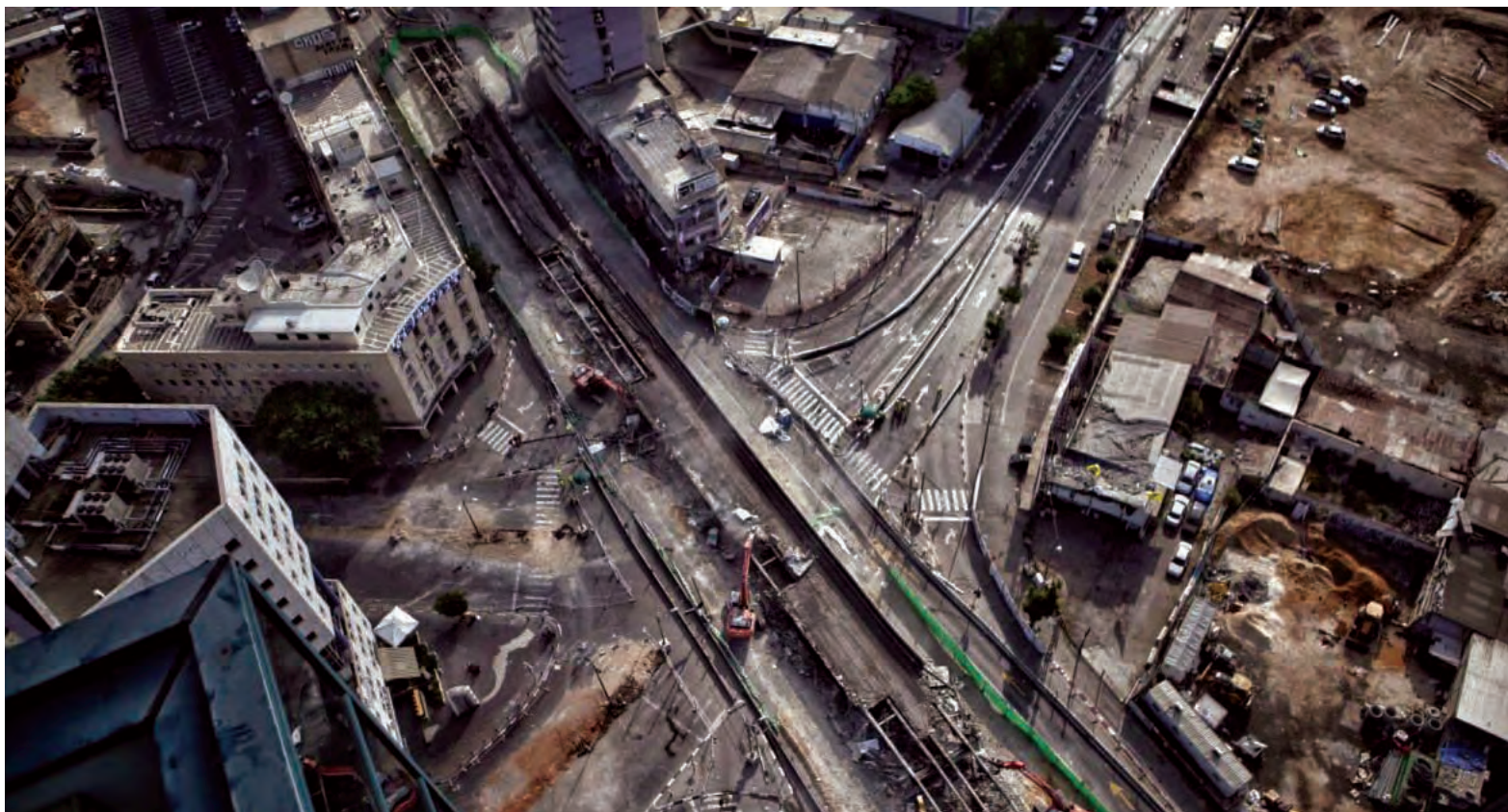
Demolition of the "Maariv" overpass to make way for the Tel-Aviv light railway station there and an underpass to replace it.
