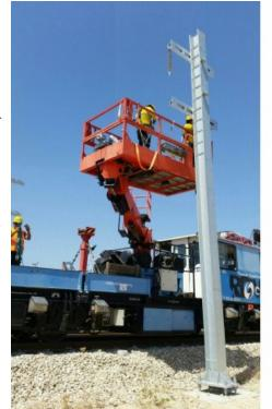
Some of the first electrification masts erected on the A1 route near Latrun in early September.
