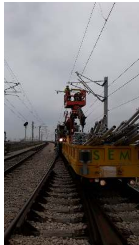
• Catenary repair works on the catenary performed by S.E.M.I. (Photo courtesy of Matan Berkovich, IR Press office.)
