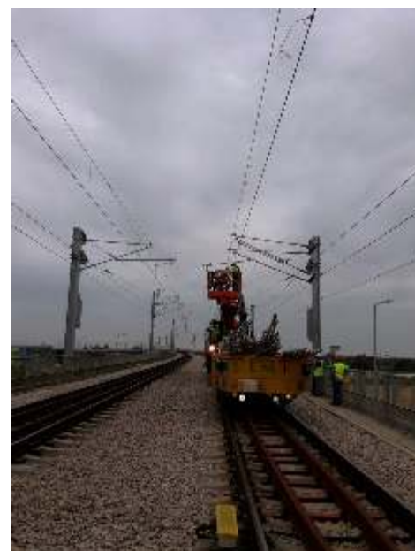
• Catenary repair works on the catenary performed by S.E.M.I. (Photo courtesy of Matan Berkovich, IR Press office.)
