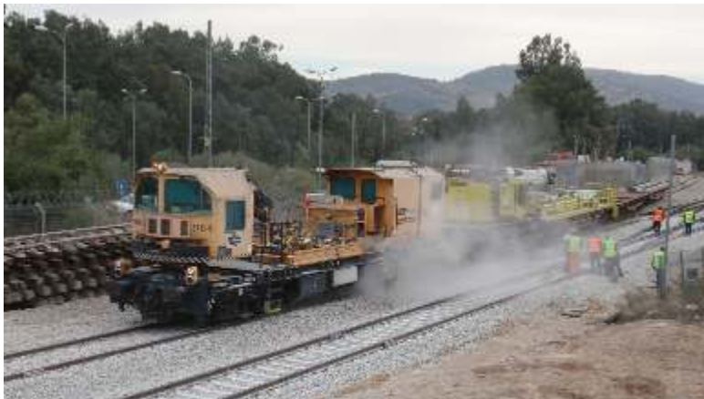
• Trackworks and turnout replacement at Beit Shemesh, 22.11.2019. (Photos Aharon Gazit)
