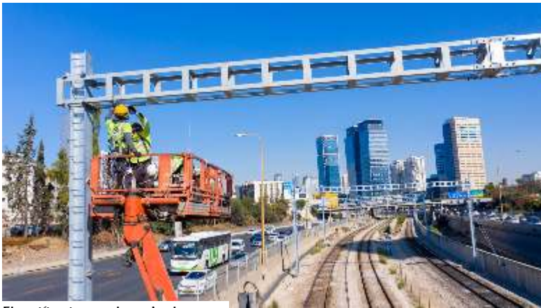
Electrification work on Ayalon.
