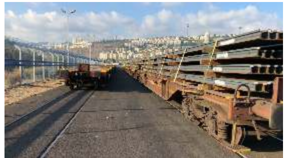
• New Rails unloaded and placed on bogie flat wagons at the Haifa Port. (Photos: Courtesy Matan Berkovich, IR)
