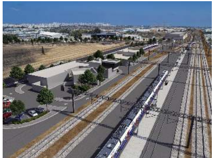
• Aerial views of new Ashkelon depot.
