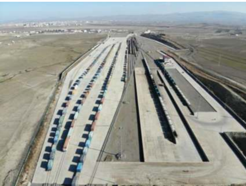
• . The new freight terminal at Kars.
