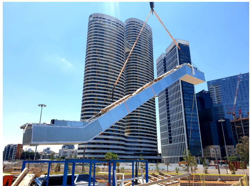
Escalator being installed in a Tel Aviv underground station. (Steve Sattler)
