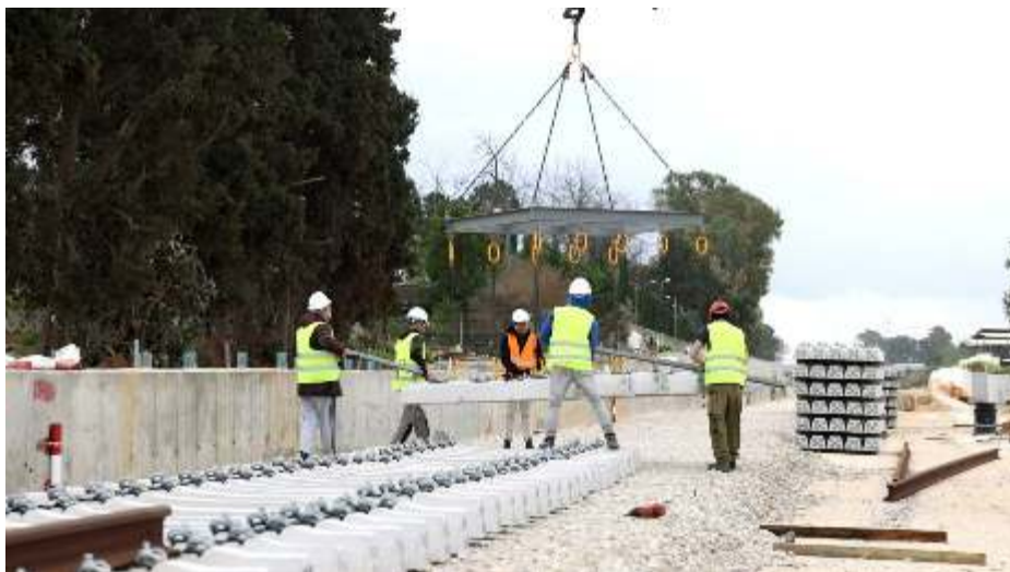
• rack laying near Hadera East. Credit for pictures: Israel Roads.
