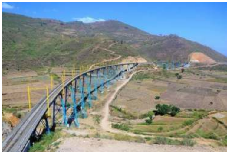
• New viaduct, in Ethiopia
