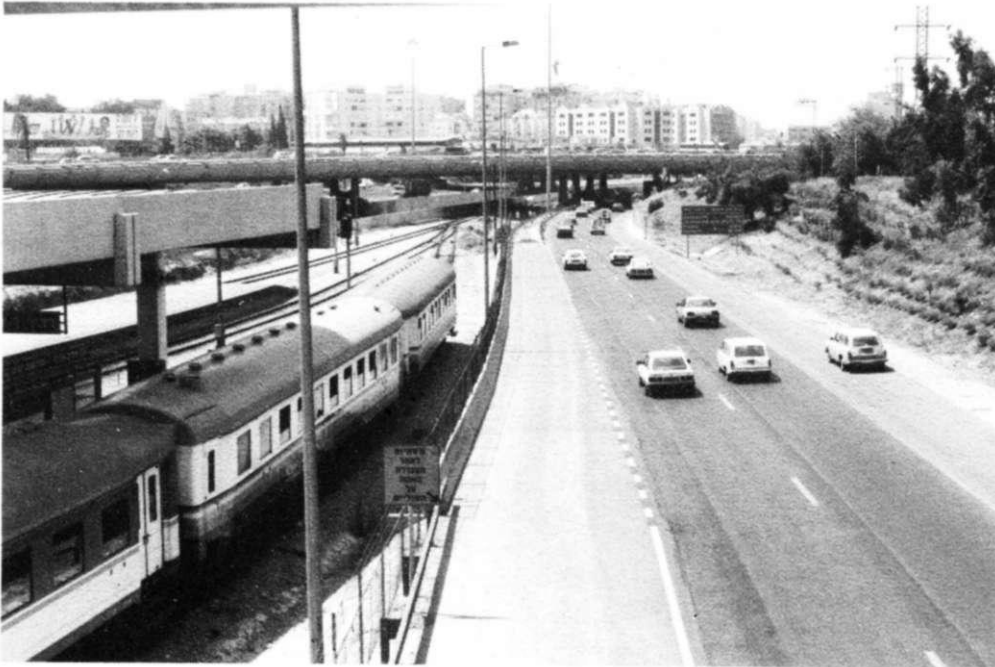
18: 3 : A look at Tel Aviv Merkaz station whilst it was still a terminus ! By the time this issue is published it could well be a through station. Looking south along the Ayalon roadway from the footbridge connecting the 'old' and the new* stations at Tel Aviv Merkaz, in July 1991; the four platform lines converge into a single headshunt, where double track will soon lead on.
