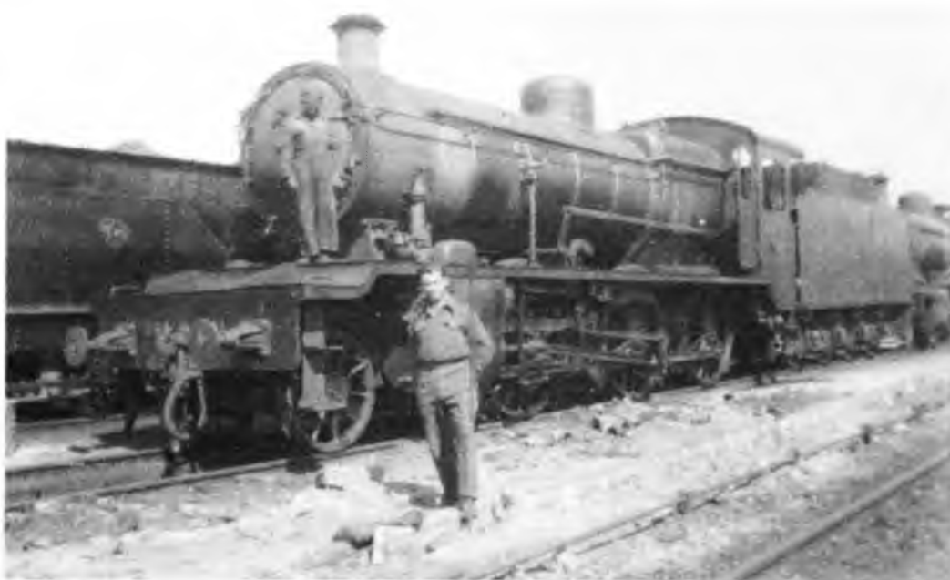
34:18: ESR 2-6-0 No. 594 - probably at Cairo. (Photo: Bert Dyke).
