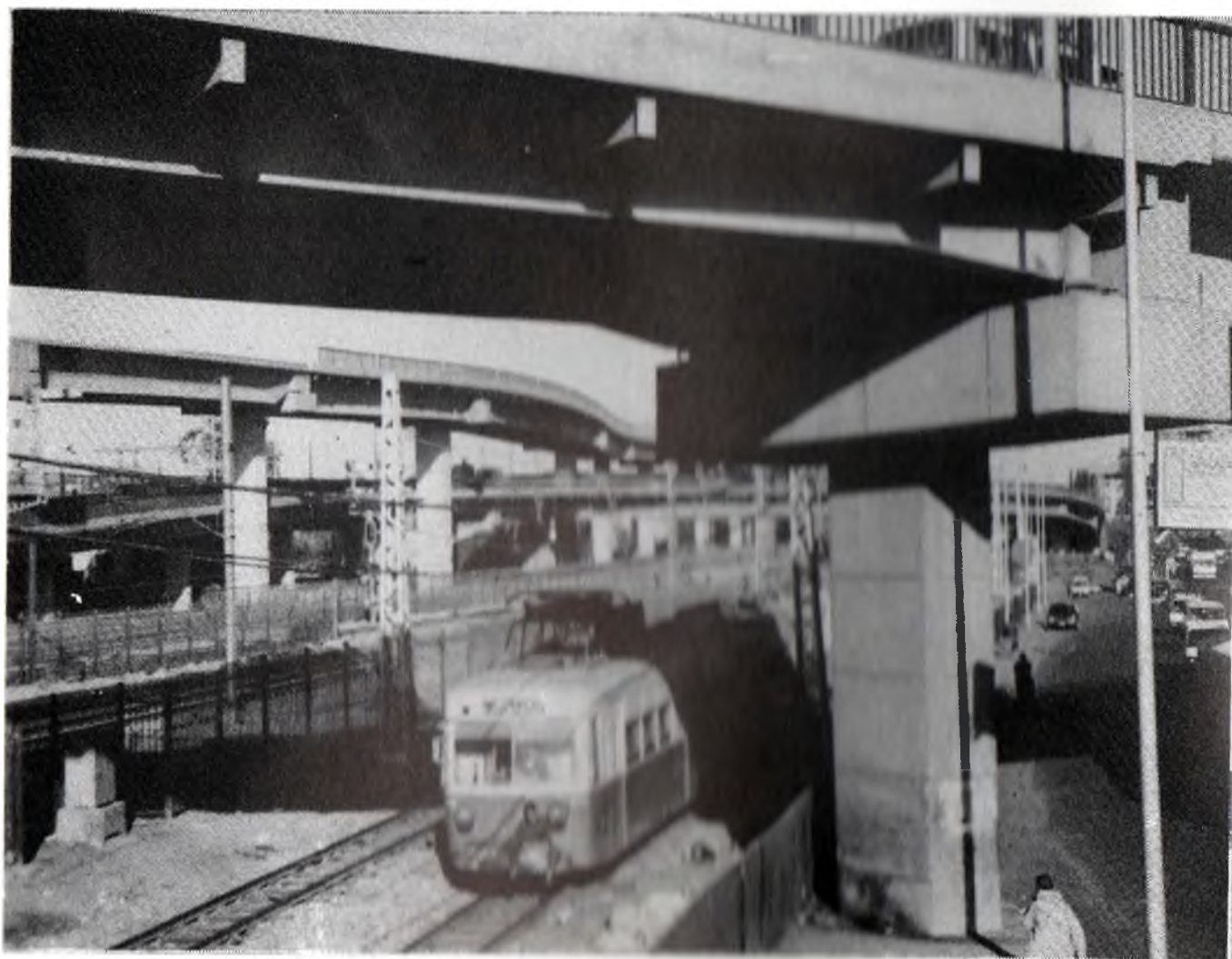
Heliopolis Metro near Ghamra Station, Cairo. 11/1/97. (Photo: Andy Wilson).
