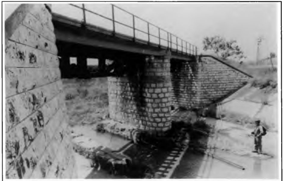
Photo 1: The latter-day 'London Bridge' looking south. Note what may be an old pier base between the central pier and nearest abutment. The WW1 2ft. 6in. line would probably have crossed the Wadi Beit Arif just beyond this bridge. (This and all photos by Paul Cotterell, 1997.)
