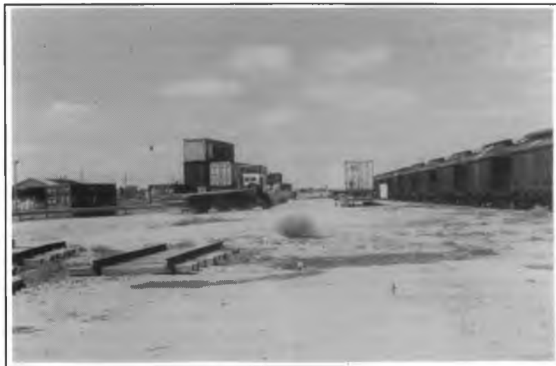
View of the container terminal at Beer Sheba Tzafon, looking north towards the passenger station: On the right, stored wagons, in the centre, lorry bringing container for loading, behind the container at left can be seen the MTR workshops building. 13/3/2000.
