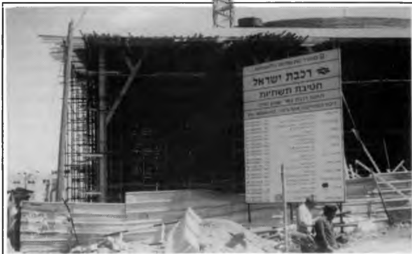
Beer Sheba Central new station under construction. 13/3/2000.
