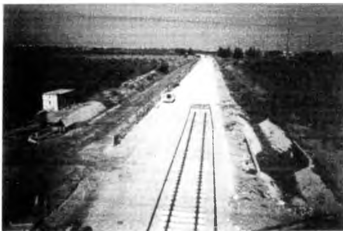
The line towards Kfar Sava under construction. Jan. 2002.
