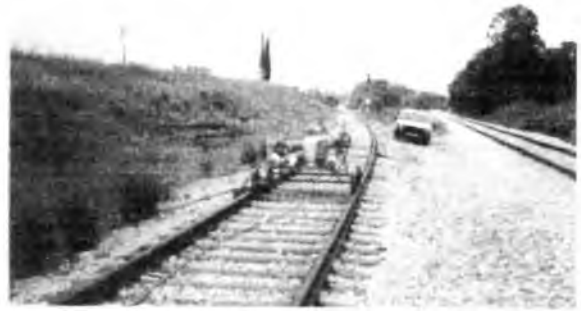
Na'an junction, looking south. The track on the left, the old line to Jerusalem, is being dismantled; the upgraded line on the right is that to Beer Sheba. April 2002.
