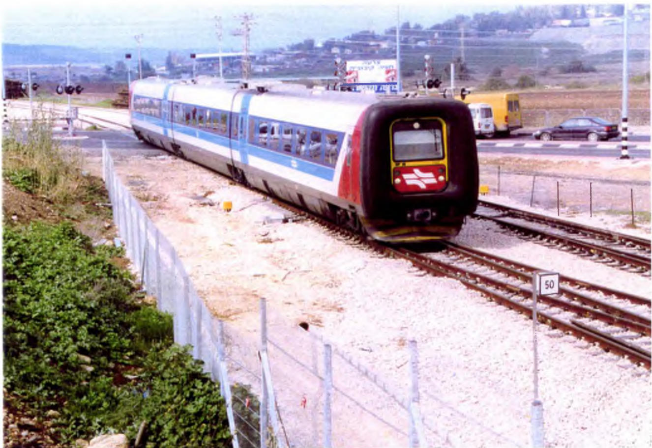
64:1. IC3 Unit 7027 approaches Beit Shemesh from the west, over the widened level crossing and approaching the pointwork for the new station, at Km. 50. 6th. Feb. 2004.
