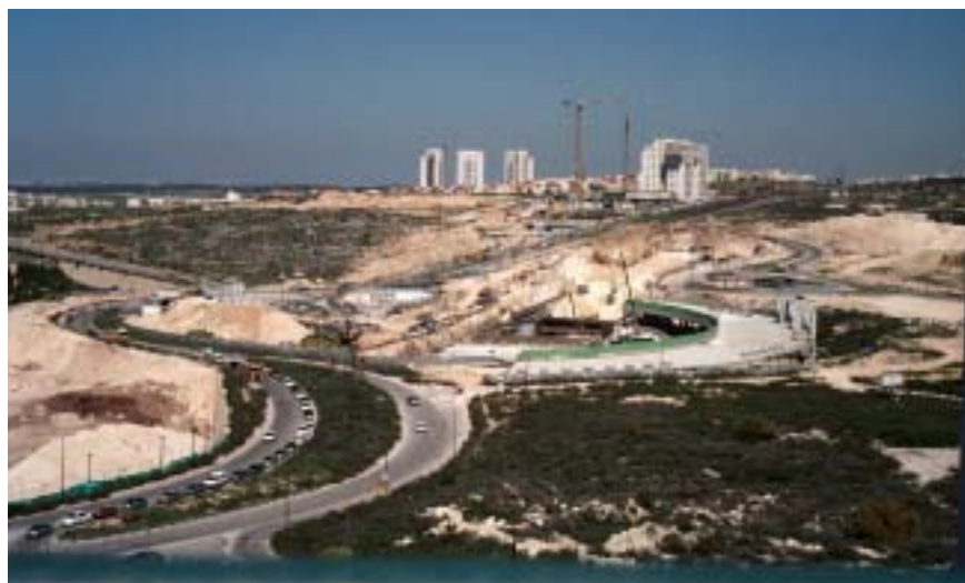
69:15 Excavation works for the Modi'in Central railway station can clearly be seen in the center of the picture Picture from A Gazit
