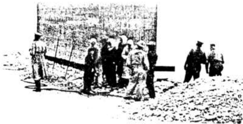
Taking the line around this steep headland, the railway engineers had to build a sea wall at a point where they had no direct access to the base of the cliff. Concrete blocks varying from 15 to 100 tons in weight were cast on the rock ledges and were tipped into the sea far below, as shown in these three pictures. When sea level was reached, men were lowered by crane down the vertical cliff to complete the work.
