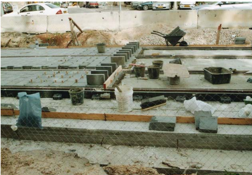
84:03/3 Surface Work Jaffa Road Feb 09
