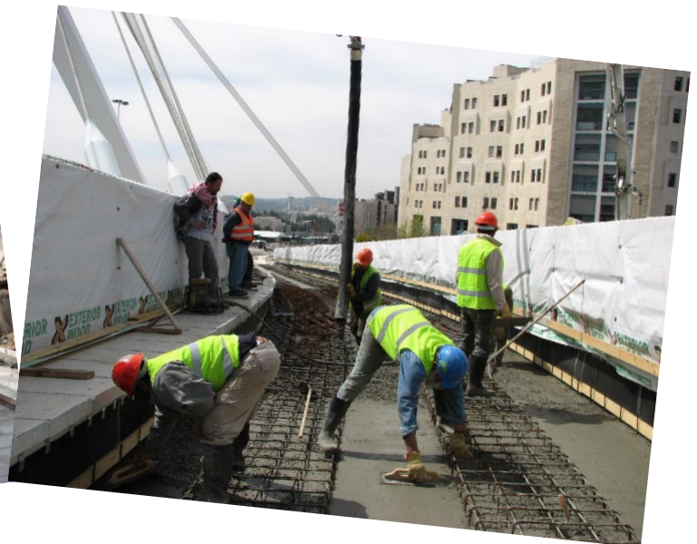
Lower right: Casting concrete on the Calatrava bridge of the Jerusalem LRV Red Line, as part of track laying; source--CityPass
