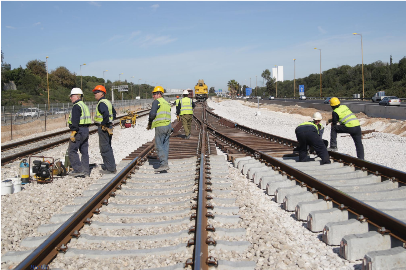
Above: Re-laying pointwork at Tel Barukh junction, Tel Aviv. Aharon Gazit.
