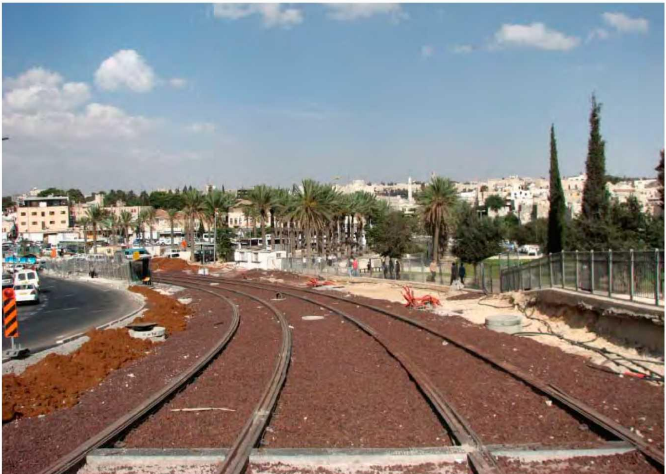
Track laying and track laid on the Jerusalem 'Red Line' LRV route, as at November 2009. (Source: CityPass.)
