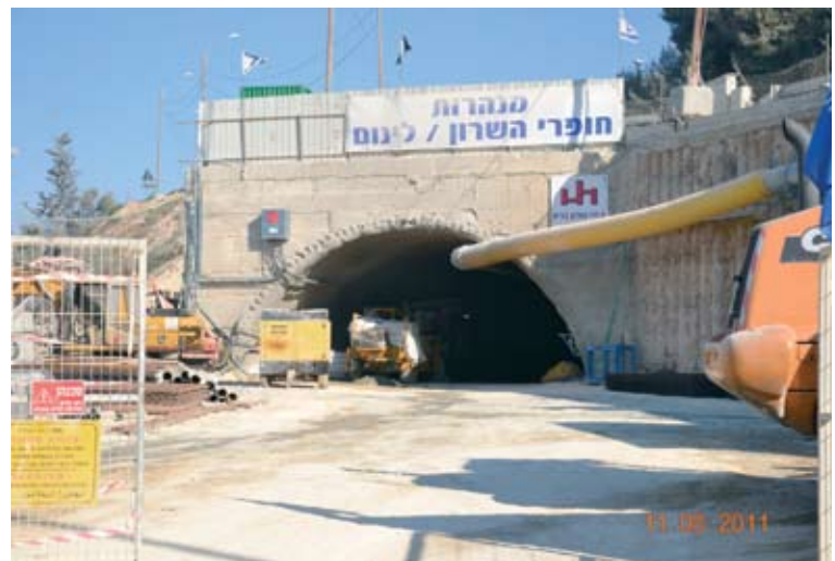
Tunnel Portals, sealing within the tunnel, and a Forming Machine.
